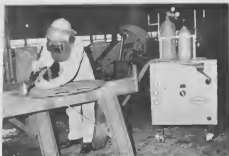
A welder here shows how he can cut out circles from a steel plate easily and effortlessly with the new Plasma-Arc cutting machine. At right, a group of welders and boilermakers are shown during a training session in the welding shops where demonstrations were given on the use of the equipment. In center, is Philip de Souza, instructor of the course.
